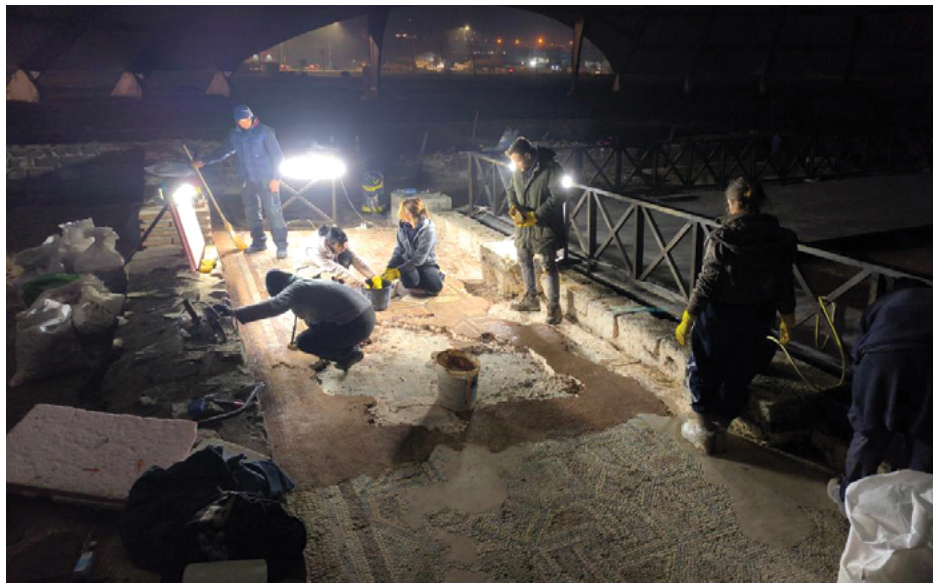
The process of mosaic grouting (photo Branko Radović)
