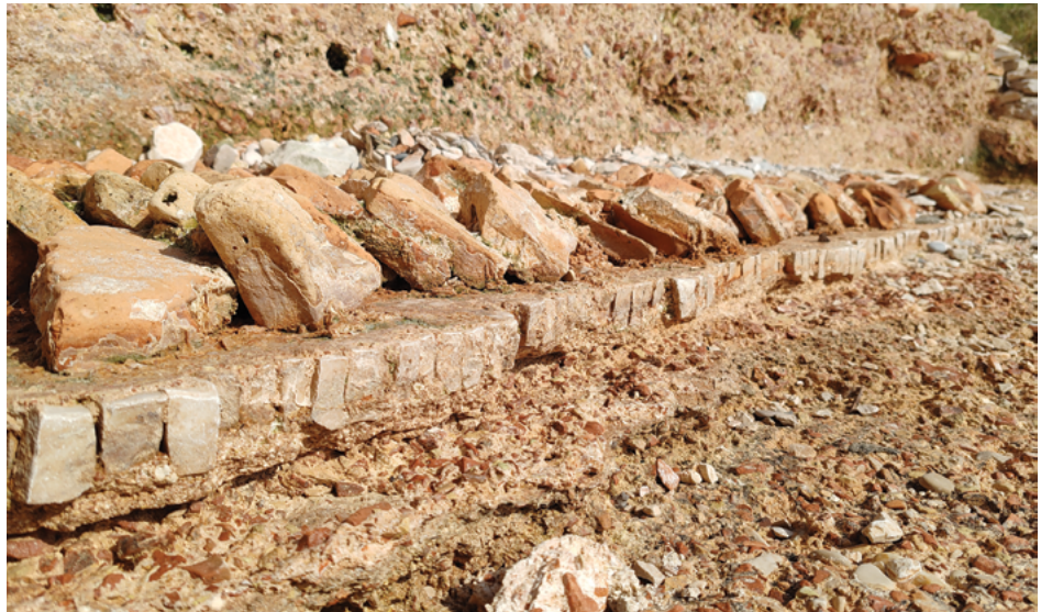
Detail of the floor layers in the cistern of Lovrečica (photo Matko Kezele)
