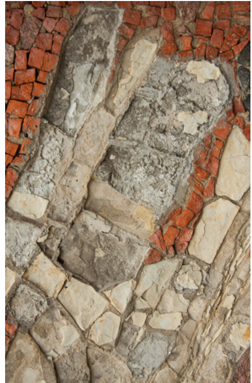
Detail of marlstone degradation (Archive of the Faculty of Restoration, University of Pardubice, Czech Republic)
