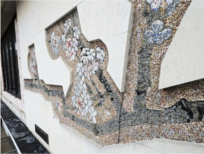
Example of a glass mosaic artwork covered due to façade insulation (ETICS intervention), Děčín, Czech Republic (photo Magdalena Kracík Štorkánová)
