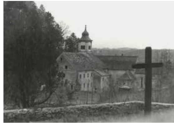
→ 46 Studenice – samostan dominikank
