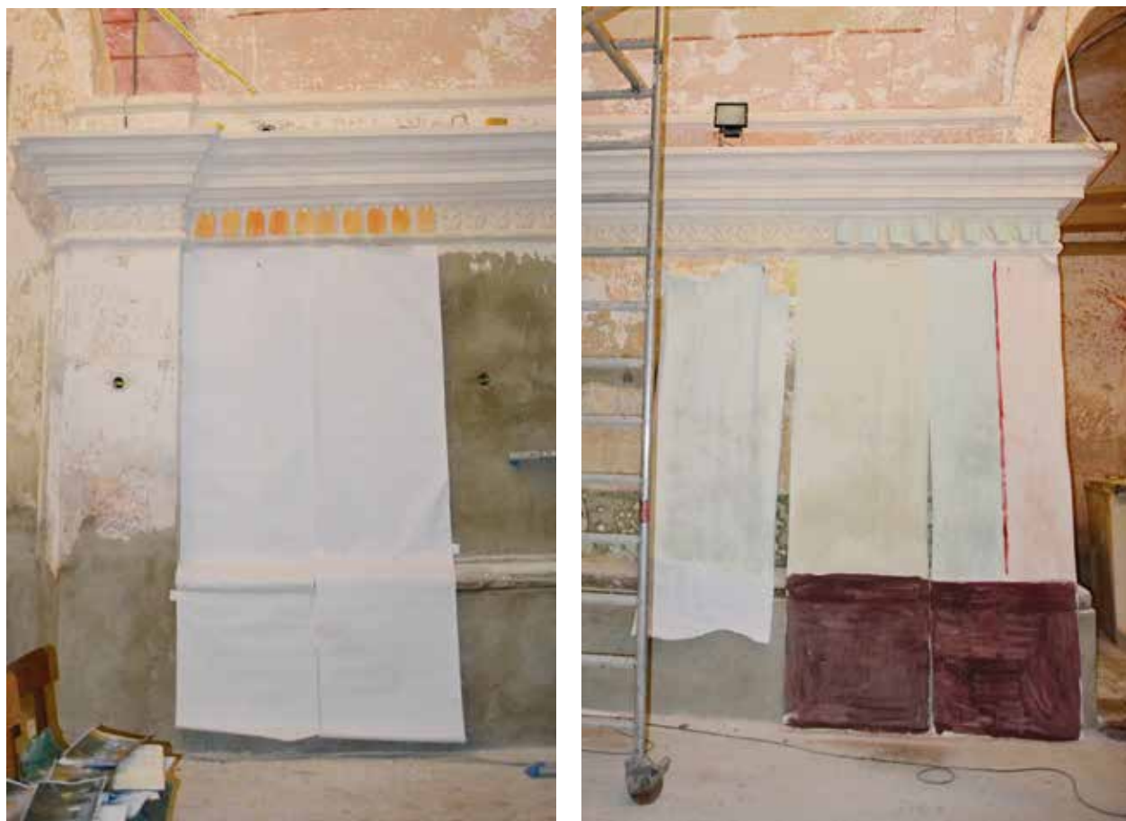
Figs. 1a, 1b: An example of a suggested painting of walls with the presentation of different phases of colour coating in St James's Church in Ledine.
