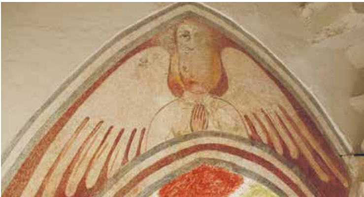
Fig. 1a: The wall painting and the outline of the angel in the presbytery of the St Nicholas's Church in Kred are reconstructed in short lines to present the original extent of the Gothic presbytery walls and their optical conclusion at the top. The fragment of the head of the Baroque angel is retouched and included in the Gothic layer. Because of the intertwining of the three layers, this solution was deemed best out of all the possible (detachment, covering or division of layers by levels or in another optical manner), since the face placed inside the Gothic painting is the least obtrusive.
