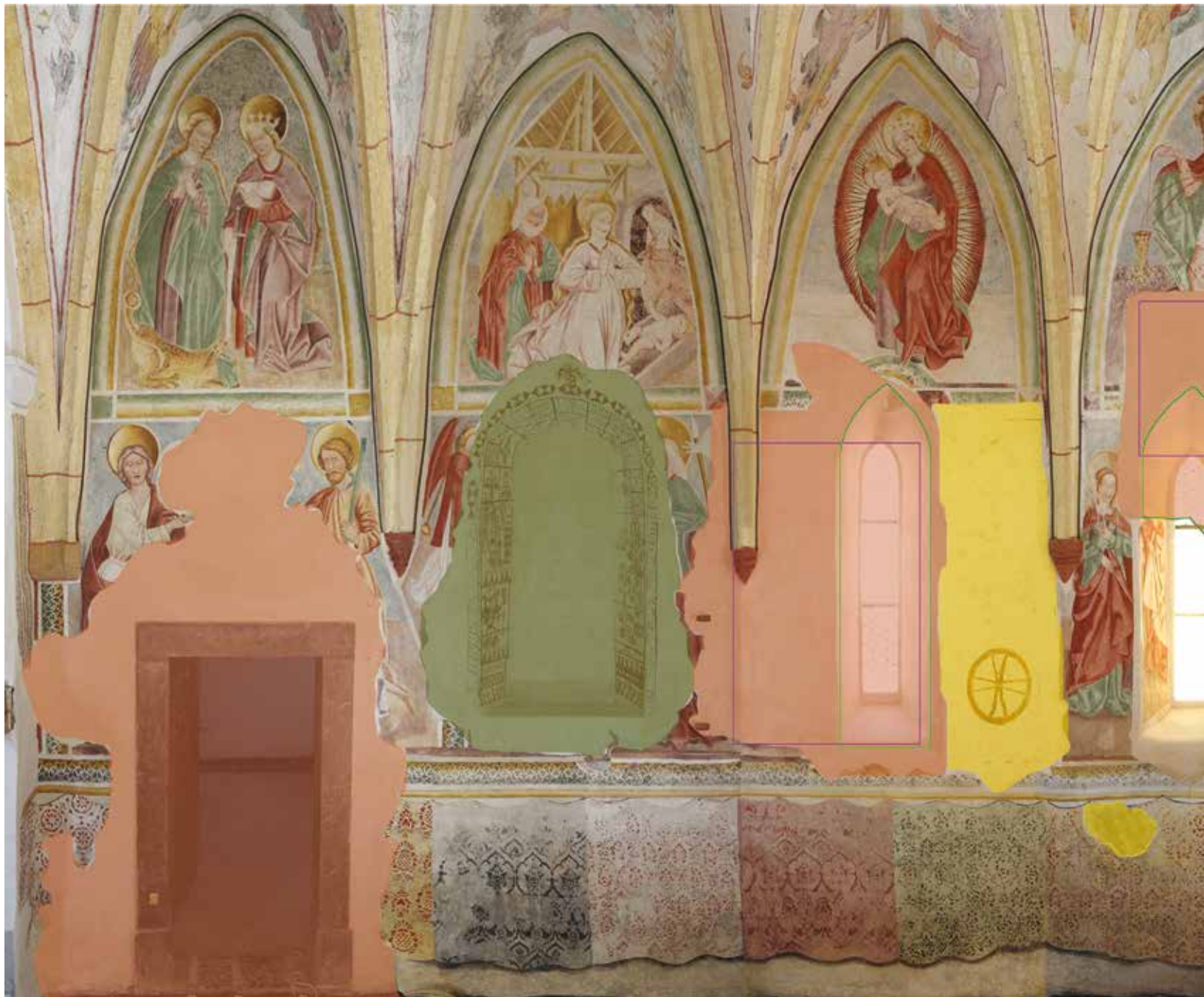
Fig. 6: Different levels and treatments of the plaster relay the historical sequence of the paintings, reconstructions, and damage as can be seen in the orthophoto of the painting from the presbytery of St Cantianus in Vrzdence with the outline and the markings of the damage and reconstructions.
