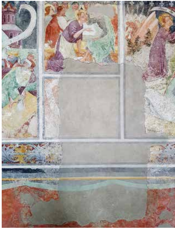
Fig. 12: The big losses in the Church of St Andrew in Thörl–Maglern (Vrata–Megvarje) are filled with toned plaster on which architectonic division is painted.
