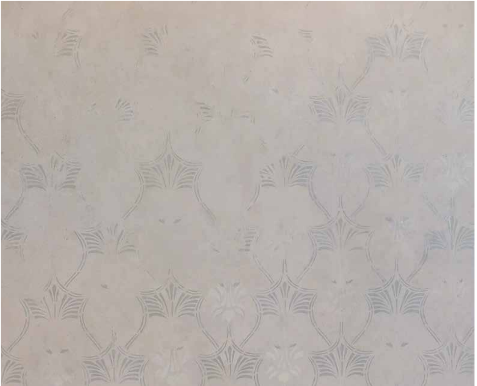
Fig. 5: On the less preserved areas of the paintings, the background is firstly tonally treated as can be seen in the example from the Švicarija, located at Pod turnom 4 in Ljubljana (2016–2017). Such a surface is then ready for the reconstruction of the missing areas of the pattern.
