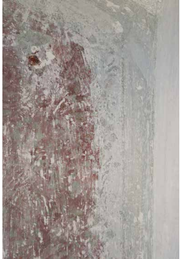
Fig. 2: Only a couple of details, discovered while meticulously uncovering the secondary layers, correctly revealed a green pattern on a lighter grey-green background.
