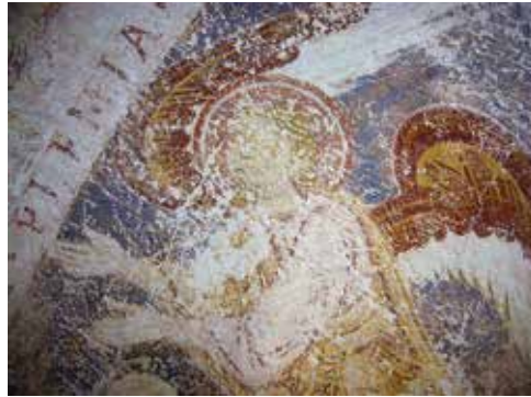
Fig. 2b: A detail of the wall paintings in the north chancel of the presbytery, uncovered in 1897, not restored yet heavily damaged by uncovering.
