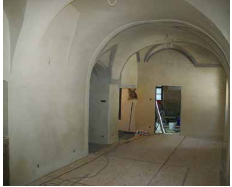
Fig. 4: The state of the same room after the reconstruction of lime plasters and the finished puttying of the original surfaces. Preparatory limewash has already been made.
