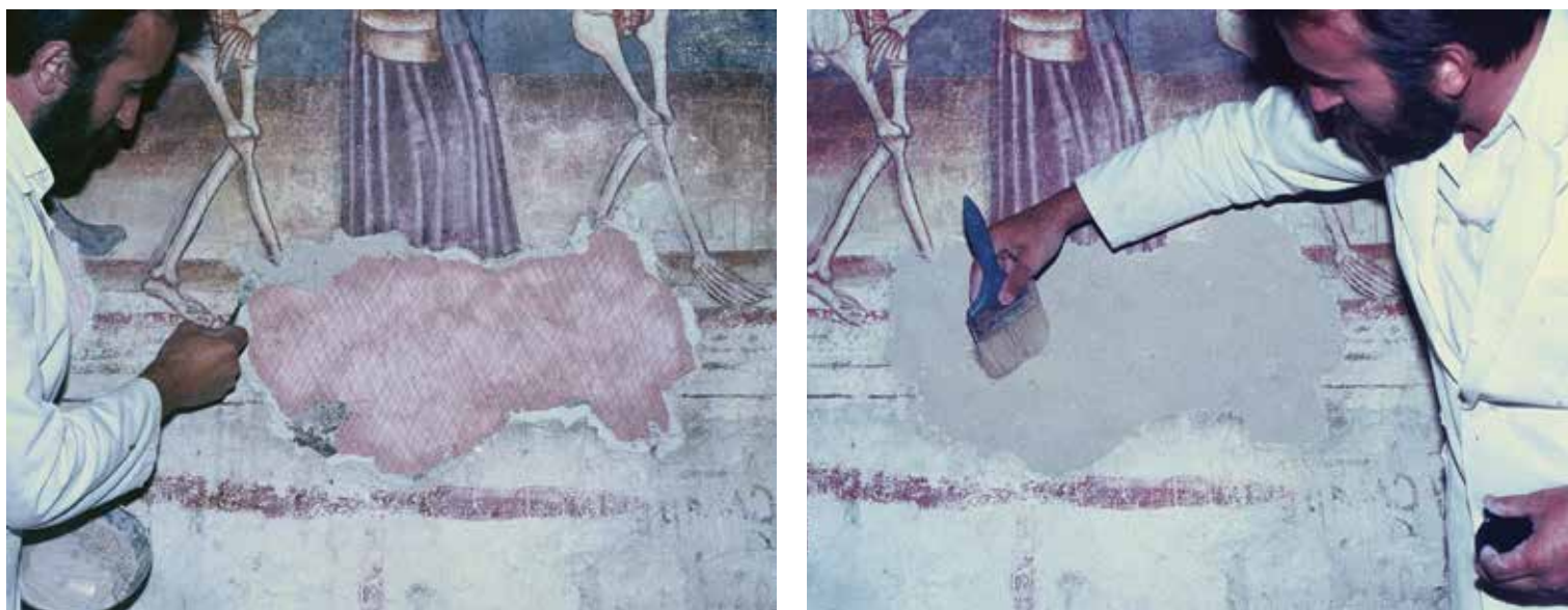
Figs. 5a, 5b: Left: a greater loss on the Hrastovlje Danse Macabre by John of Kastav (1490) treated with rough red plaster. Right: treated with smooth decorative plaster applied on top of the red.
