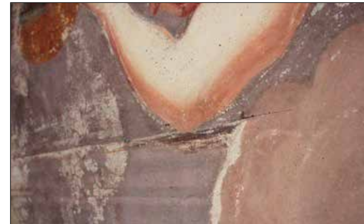
Figure 141: Rare auxiliary lines, cut directly into the fresh plaster, without cartoons, were noticed when mapping out the architecture, which served as orientation points onto which the red preparatory drawing leaned.
