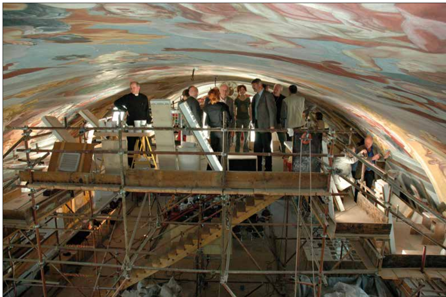
Figure 24: Relevant committees view the last stage of restoration work (22 May 2006).
