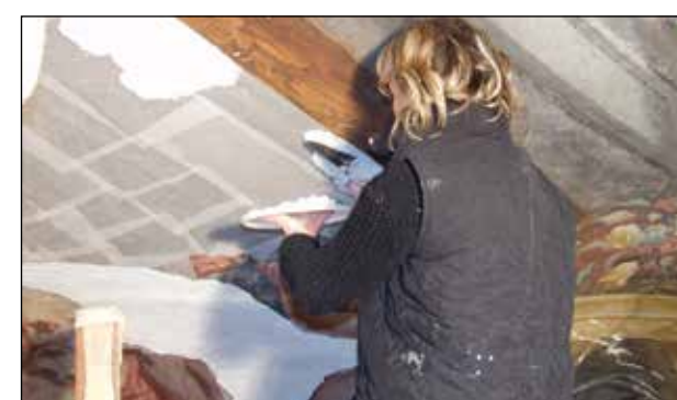
Figure 12: Beginning of chemical cleaning (25 February 2004).
