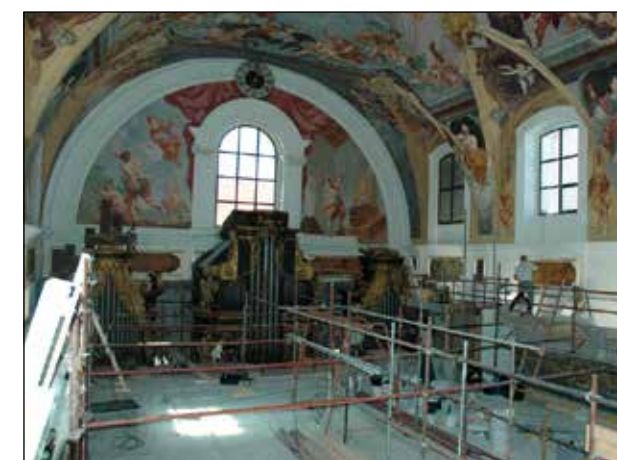
Figure 25: Finishing touches after removal of restoration scaffolding (31 August 2006).
