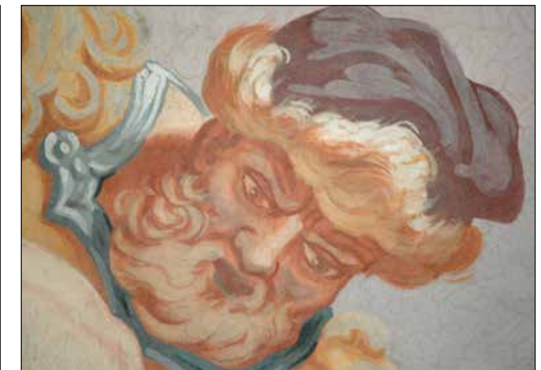
Figure 228: Condition after the renovation – the cracks are less noticeable after cleaning and retouching.
