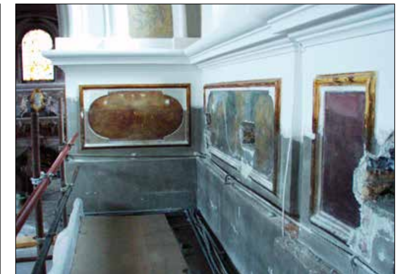
Figure 238: Visible openings into which the anchor ties of the scaffold were inserted and the difference between the cleaned and uncleaned surfaces.
