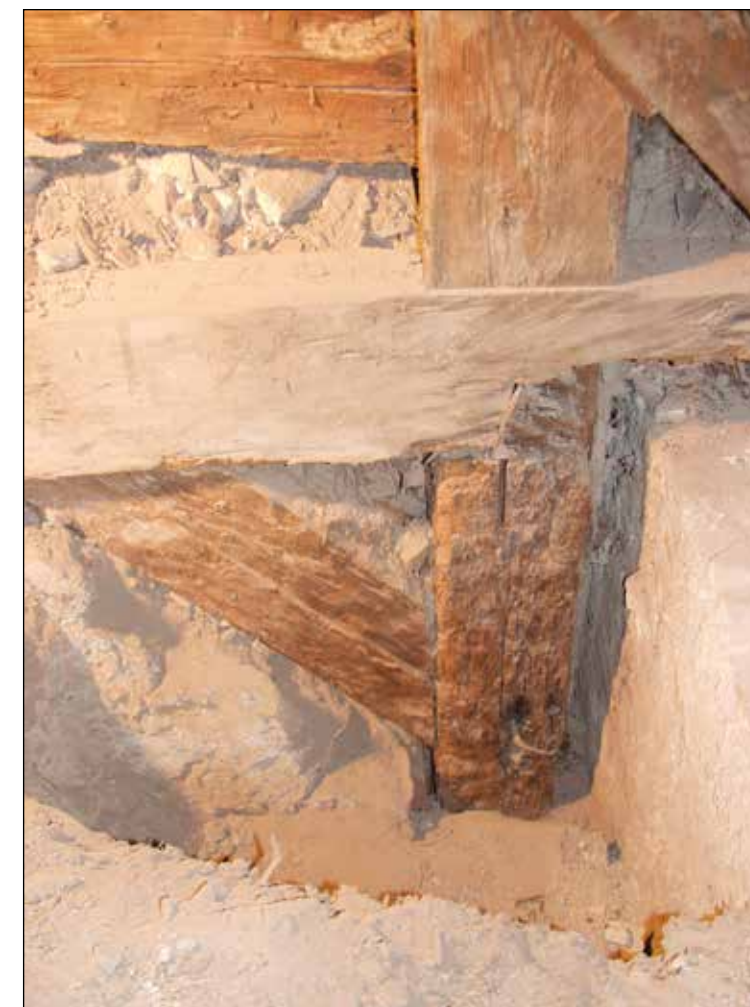
Figure 42: The anchoring in the roofing construction.
