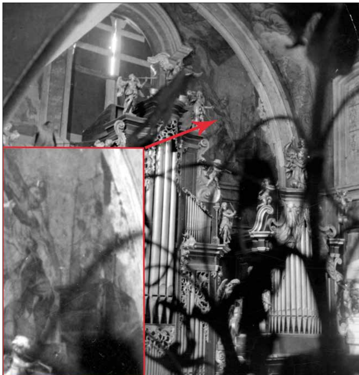
Figure 14a: The damage on the western wall was caused by the 1895 earthquake and by the restorations of the western gable and the organ. Jebračič's reconstruction of Nicholas's head can be seen on France Stele's photograph of the organ from 1952.
