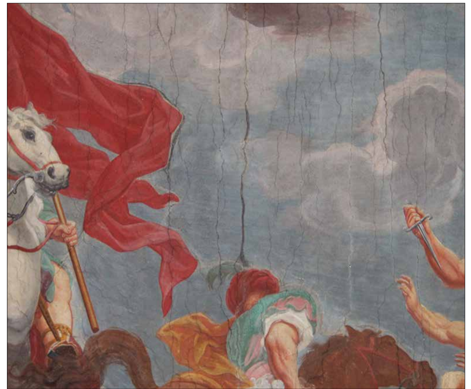
Figure 203: The region above the organ with the thickest network of cracks; in the middle and to the left along the red drapery, darkened retouches from a previous restoration treatment.
