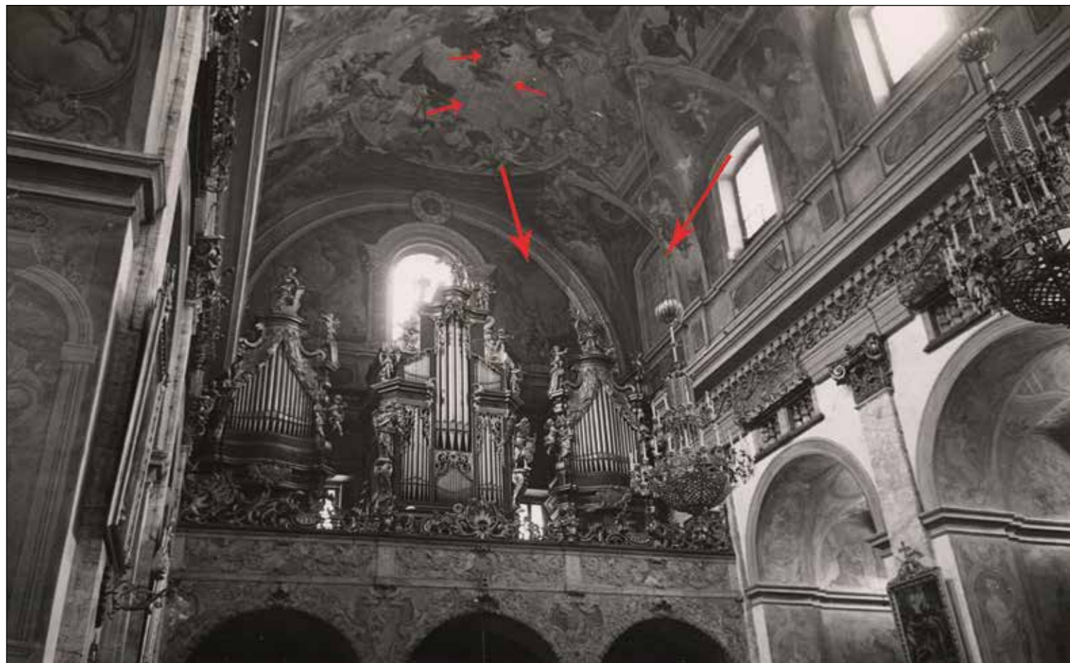
Figure 8b: A shot of the interior looking north-westwards, perhaps taken by Peter Železnik, with visible damages in the area adjacent to the bell tower and the decorative painting on the blind window.
