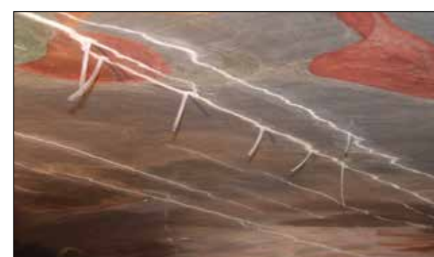
Figure 14: Inserting tubes for injecting (2 April 2004).
