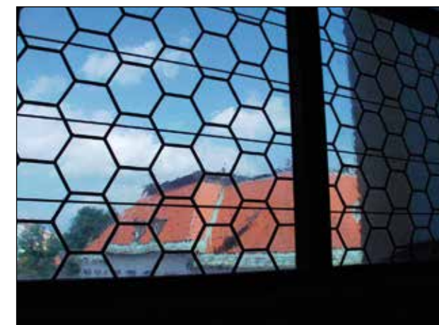
Figure 21: Installation of new stained glass (7 September 2005).
