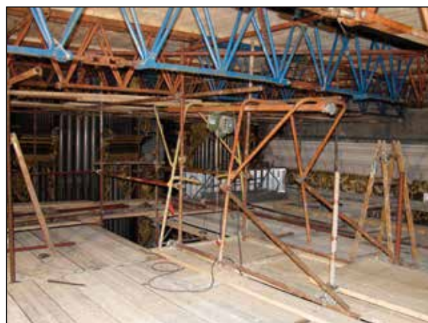
Figure 1: During construction of the restoration scaffolding (24 October 2002).
