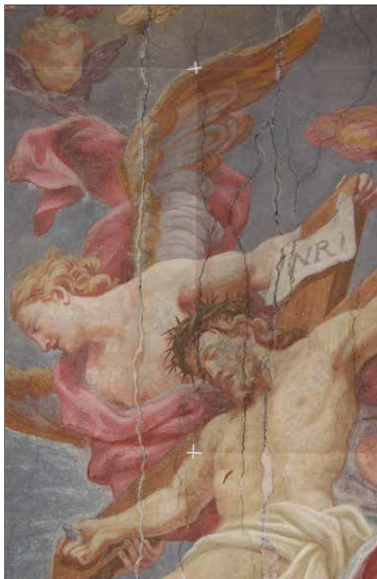
Figure 244: Condition before the renovation of the vault painting in Ljubljana Cathedral.
