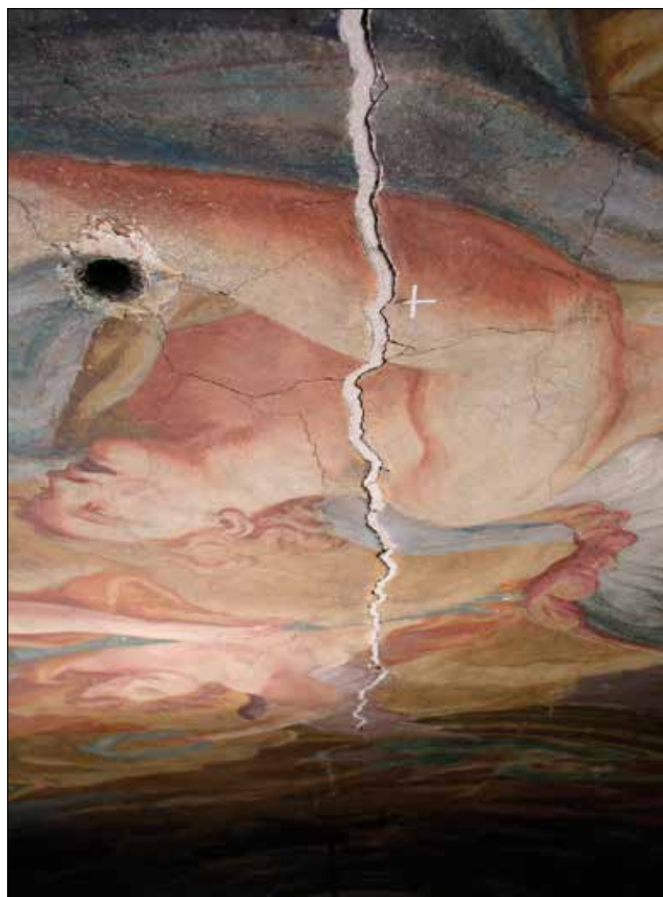
Figure 32: Condition before treatment – a new crack, next to another, once already filled crack, runs along one side and then the other.
