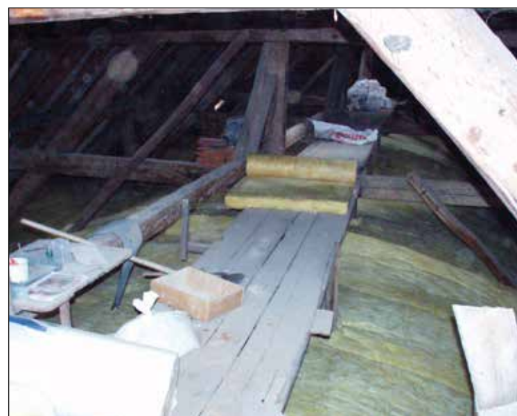
Figure 44: Applying thermal insulation to the vault.
