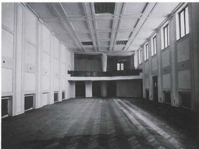
Original state of the theatre hall (Architecture Museum of Ljubljana, Plečnik Collection)
