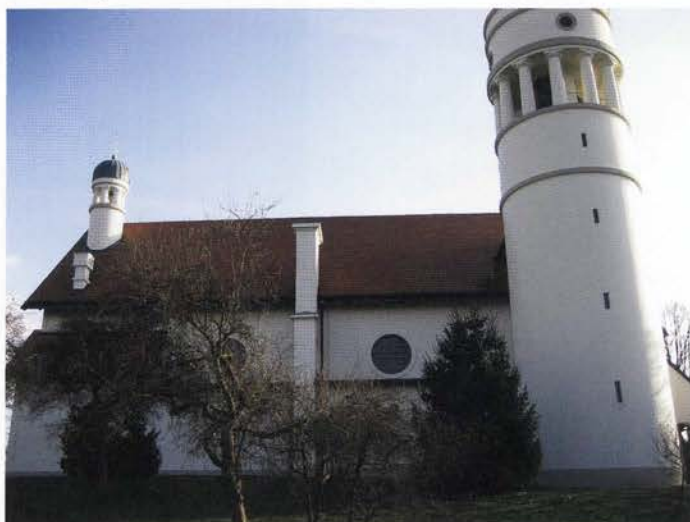
Southern façade after renovation, autumn 2006
