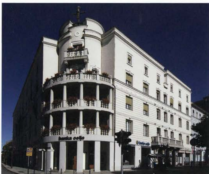
Present-day state of the connecting element in the corner of the street façades
