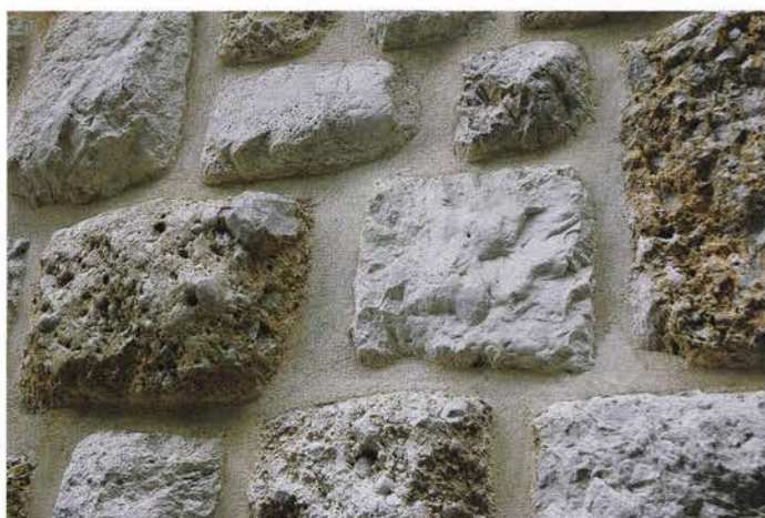
Detail of stone façade
