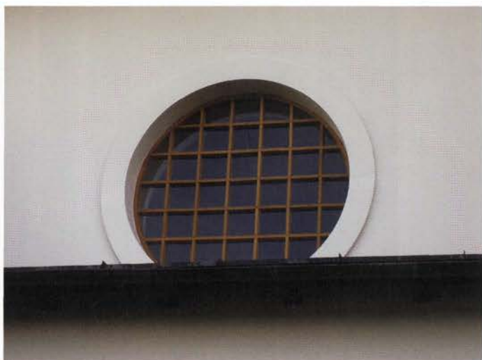
Disused windows were replaced with new ones .....
