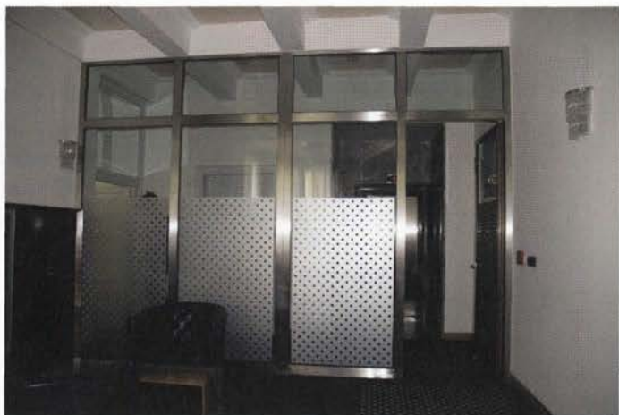
Inappropriate barrier in the corridor
