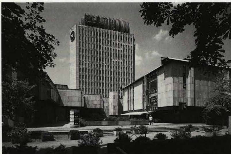
“Ravnikar endeavoured to preserve the exposed position of the two towers, therefore the extensions formed a contrast.”
