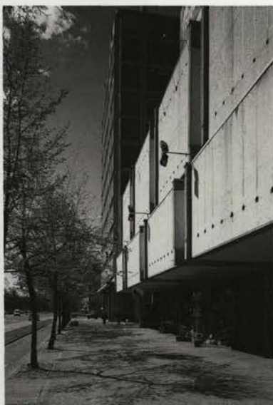
Department store ... "It is a modular layout of the so-called additive architecture, created with ferroconcrete frames with interpolated cubic bodies."
