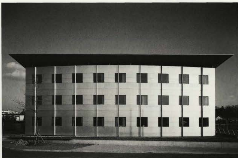
Facade of the administrative building ... "Lešnik used prefabricated metal facade panels functioning simultaneously as heating elements."
