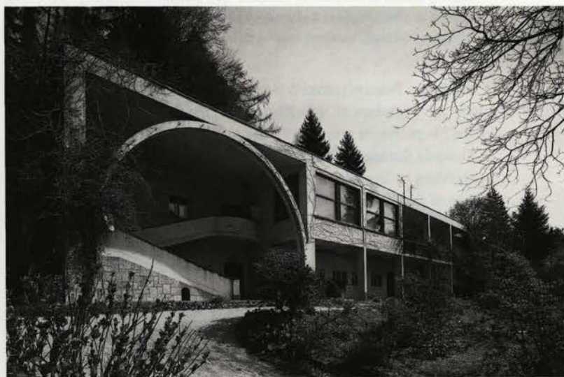
"A distinctive feature of the Oblak villa was the vestibule with the external staircase marked by a large concrete arch."
