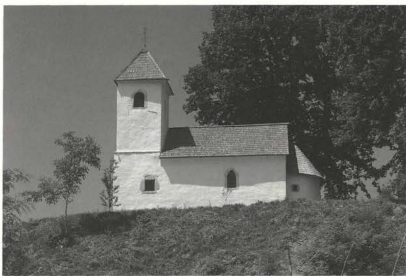
View of the church after the restoration: "The church is an important example of our heritage on account of its interesting history..."
