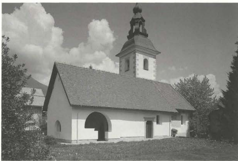
Exterior of the church: "It is hoped that the monument is now saved from further ruin as a result of the enumerated works and that some of its original freshness has been restored..."
