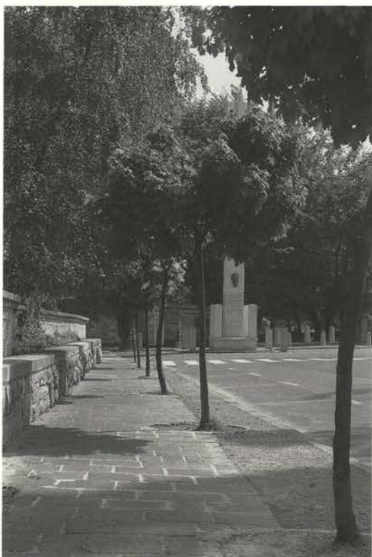
Vegova Ulica: "The walkway along the entire course of Vegova Ulica was paved with porphyry slabs and separated from the road with a sand surface planted with ball-shaped maple trees..."
