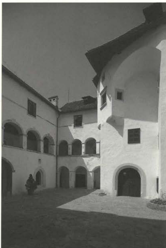
View of the renovated courtyard: "Trial boreholes made from the inside of the wall indicated the original entrance. The present semi-circular portal was built in..."
