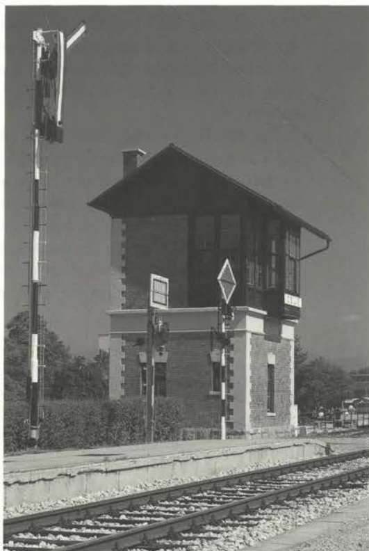
Renovated signal box: "The Southern Railway Board comprehended the new situation and granted the construction of the most advanced signal box of that time on its lines." .....
