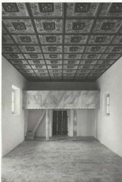
View of the renovated interior of the church: "The restoration of the coffered ceiling, dated by Dr. Nataša Golob as belonging to the period around 1680, began in 1999."
