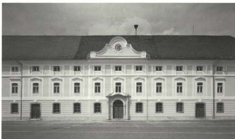
Renovated entrance wing of the manor: "Despite all transformations in the historical construction development, the Selo Manor complex has been preserved."
