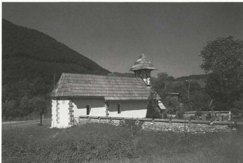
Renovated exterior of the church of St. Gilbert. "After several years of effort to preserve the church from ruin the restoration of the building was begun in 1986 by the Institute..."
