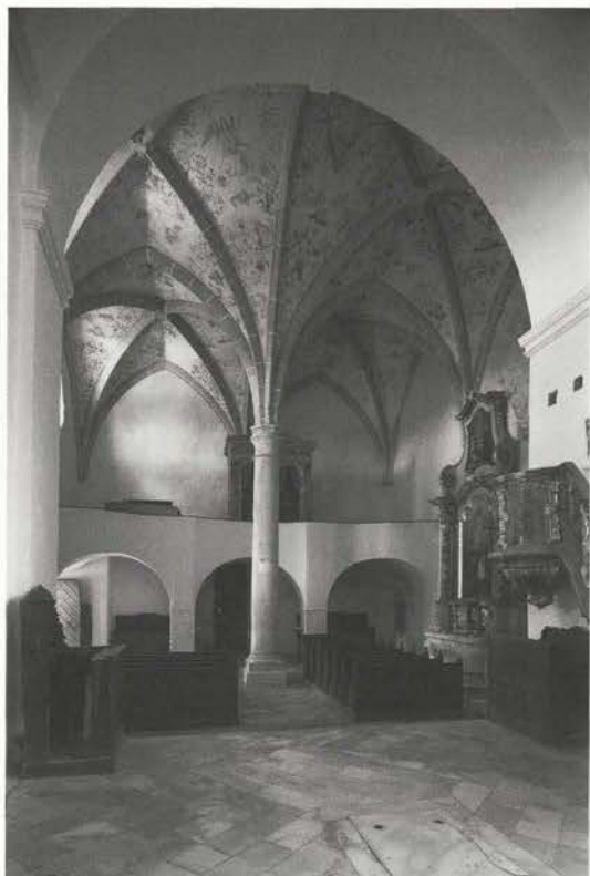
Central column with the cross vault of the nave. "Attention is drawn particularly to the central monolithic column as the bearer of the cross vault. A Roman column found in the ruins of the near-by antique settlement of Colatio was presumably used for it..."
