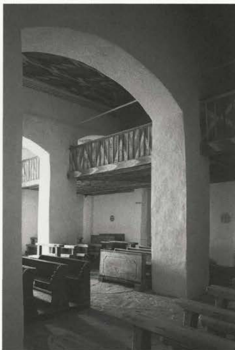
View of the renovated wooden choir. "Therefore the decision to perform the reconstruction of the entire ceiling was taken, with the exception of the choir banister and the ceiling above the choir..."
