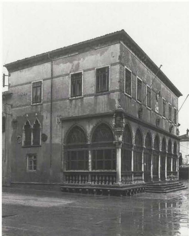
Loggia in 1935. "The adaptation was most thorough in 1846 when the Gothic arched vaults were closed by wooden frames as part of the rearrangement of the interior..."
