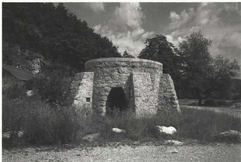
Renovated lime-kiln in Podutik. "There were usually five lime-kilns readied for operation every year. The production increased after the earthquake in Ljubljana at the end of the previous century..."
