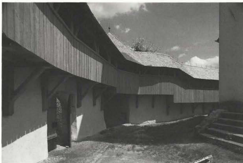
Reconstructed wooden defence parapet. "For the reconstruction of wooden elements the remnants were compared with the preserved or already renovated strongholds in Carinthia and both the rebuilt strongholds in Slovenia..."
