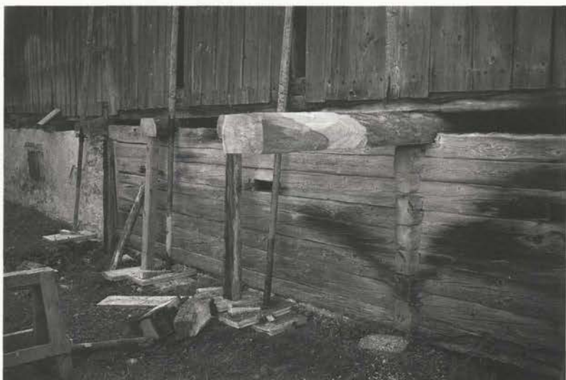
Renovation of the outhouses. "The walls of the hayloft were panelled with vertical boards fixed with wooden tacks to the beams of the supporting timber construction..."
