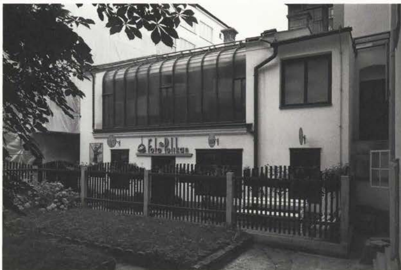
The Pelikan studio after the renovation. “...the key issue was the glazing of the studio. The dilemma was whether to insist on single-layer glazing, thus ensuring the authenticity of the historic building...”
