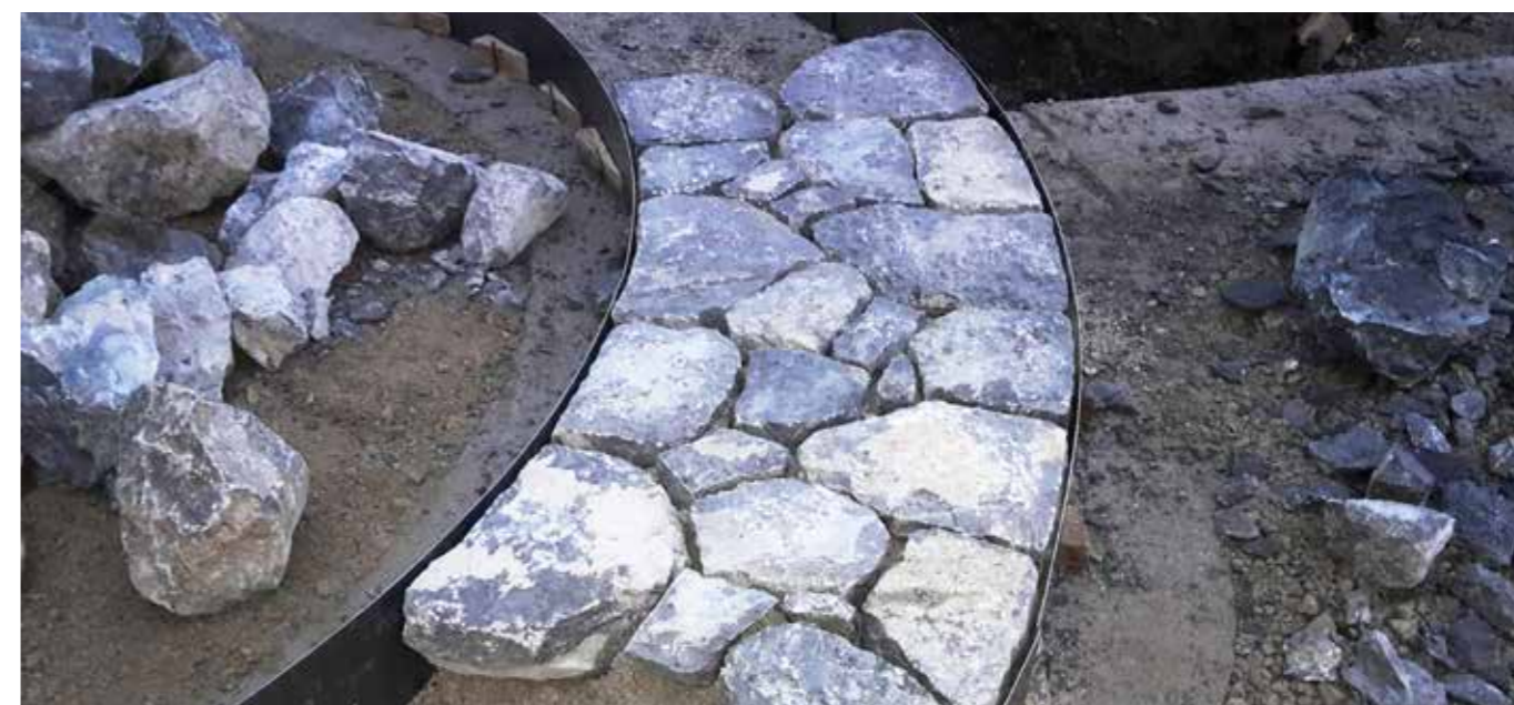
8b. Rekonstrukcija pozidave stolpa (foto: K. Udovč, ZVKDS, CPA) 8b. Reconstruction of the stonework of the tower (photo: K. Udovč, ZVKDS, CPA)
