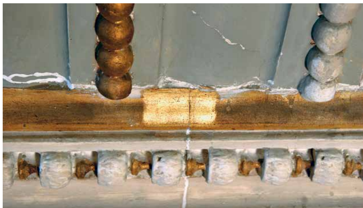
7. Poskus čiščenja originalne pozlate na štukaturah stropa (foto: Emanuela Querini) 7. Attempt at cleaning the original gilding on the stuccowork of the ceiling (photo: Emanuela Querini)
