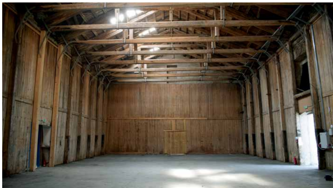
4. Notranjost 3. kampaite skladišča Monfort z lesenimi oblogami sten (foto: Ana Plestenjak) 4. Interior of bay 3 of the Monfort warehouse with wooden wall cladding. Photo: Ana Plestenjak
