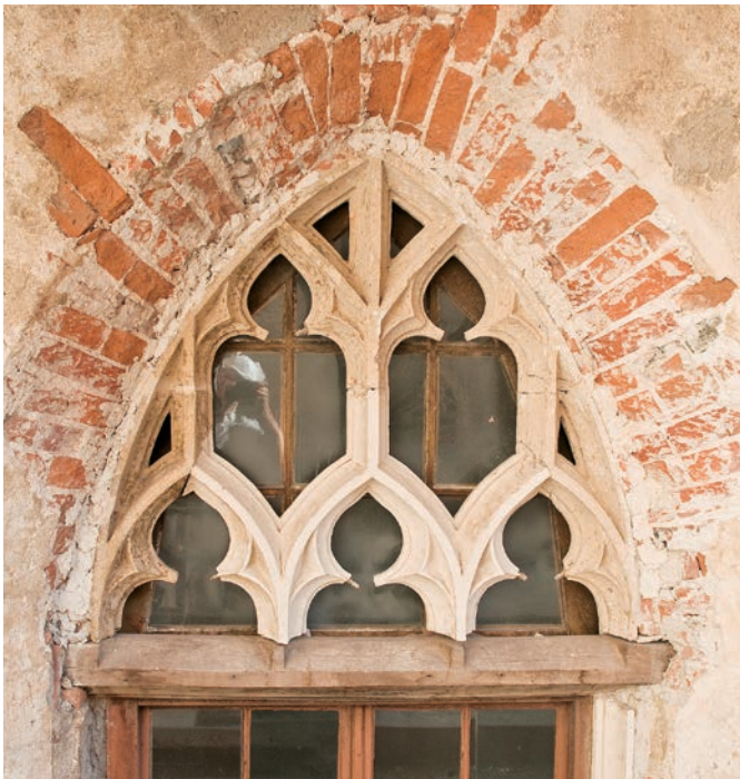
21. Ptuj, dominikanski samostan, krogovičje levega okna severnega kraka križnega hodnika med čiščenjem (foto: Robert Peskar) 21. Ptuj, Dominican monastery, tracery of the left window in the northern cloister tract during cleaning (Photo: Robert Peskar)
