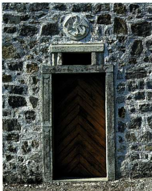
Restavrirani renesančni portal s kopijo sklepnika Restored Renaissance portal with a copy of the boss
