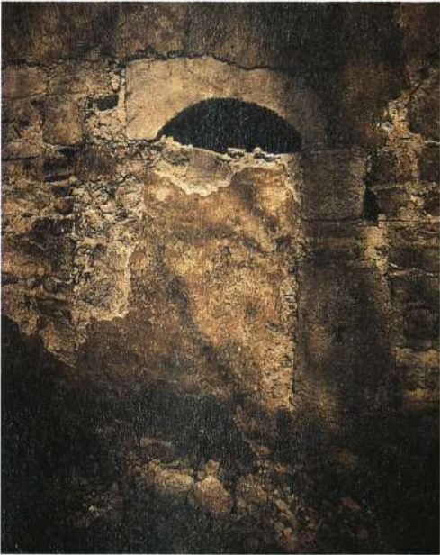
Zazidani romanski portal
