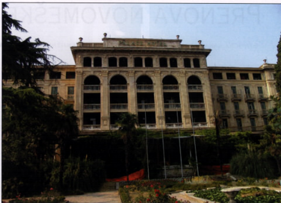
Hotel Palace pred obnovo
