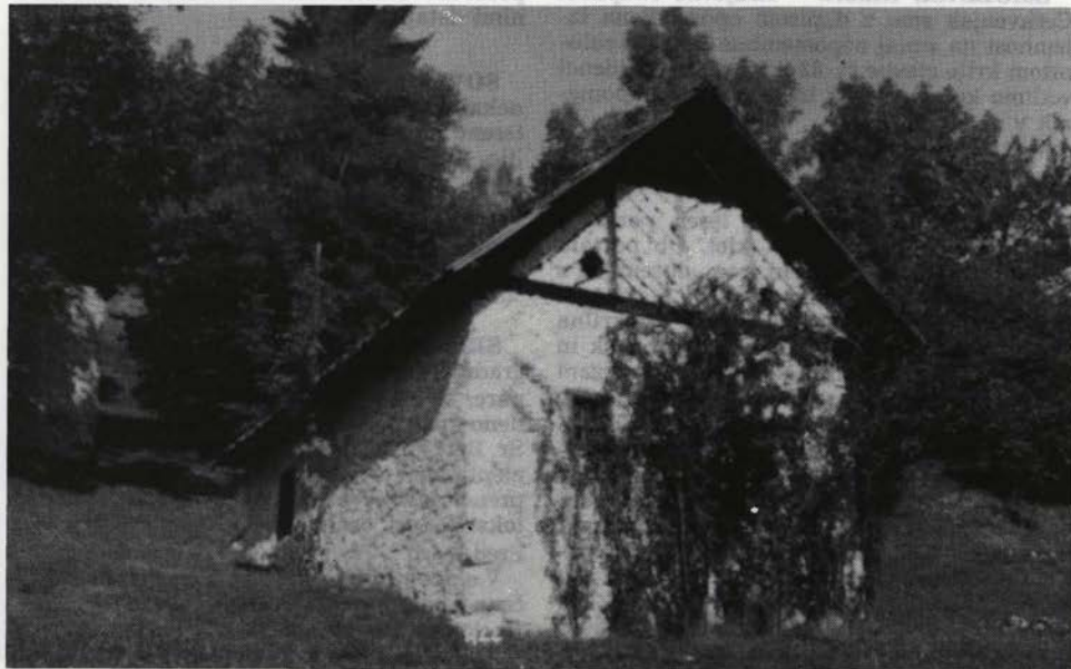
Sl. 131. Srednja vas v Bohinju, planina Šeh – dvocelični, zidani stan (lesena kritina) Fig 131. Srednja vas v/in Bohinj, Šeh – the two-celled, built lodging (wooden covering)
