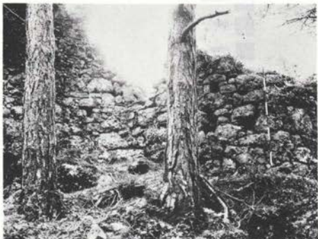
Sl. 61 Podnanos, Tabor – ruševine S zidu z delom stolpa 61. Podnanos, Tabor/Fortification – the ruins of the northern wall with part of the tower
