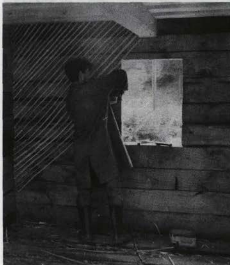
Sl. 127. Rogatec, spominski muzej – »pušňanka«, leskove palice na notranjih stenah (fotoarhiv ZVNKD Celje 1990) Fig. 127. Rogatec, open-air-museum – the typical seasonal wine-shop, hazel-tree sticks on the interior walls
