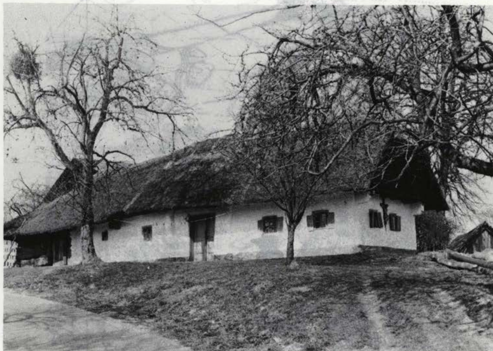
Sl. 117. Kukava 61 – značilna viničarija, cimprana, krita s slamo. V zalomljenem tlorisu je bil gospodarski del s prešo Fig. 117. Kukava 61 – the characteristic vinedresser's cottage, wooden, straw-covered; in L-shaped ground-plan had been placed the outhouse part and the wine-press
