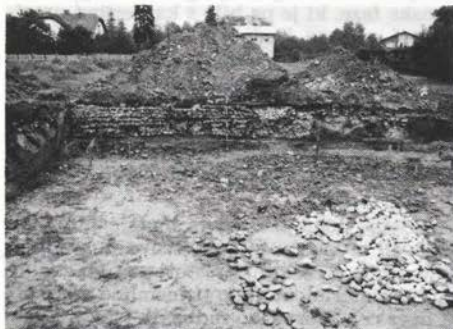
Sl. 98 Ptuj, Rozman, parc. št. 2123/1 in 2 k.o. Ptuj – pogled na severni profil z zidom in zidavo »ribje kosti« 98. Ptuj, Rozman, parcel no. 2123/1 and 2 cadastral communities Ptuj – view to the northern profile with the wall and building technique "fish bone".
