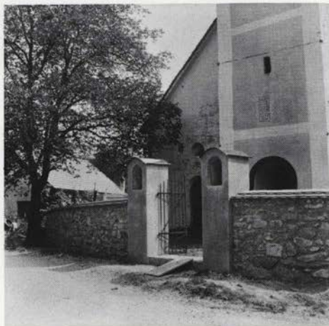
Sl. 132 Zavoglje – pokopališki zid pred in po obnovi Fig. 132 Zavoglje – the cemetery wall before and after renewal
