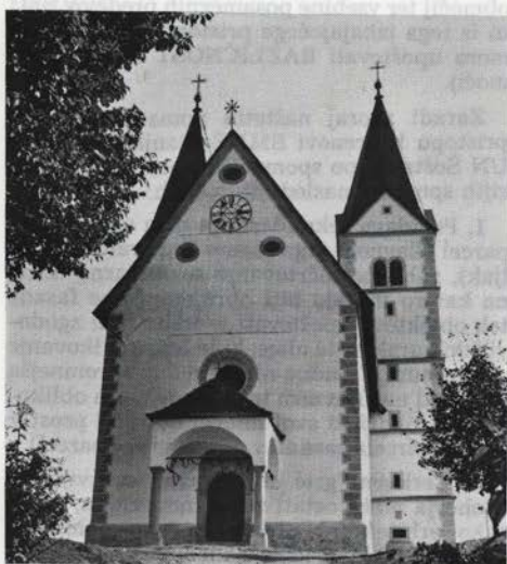
Sl. 128 Šmihel – obnovljena zunanjsčina Fig. 128 Šmihel – renewed church
