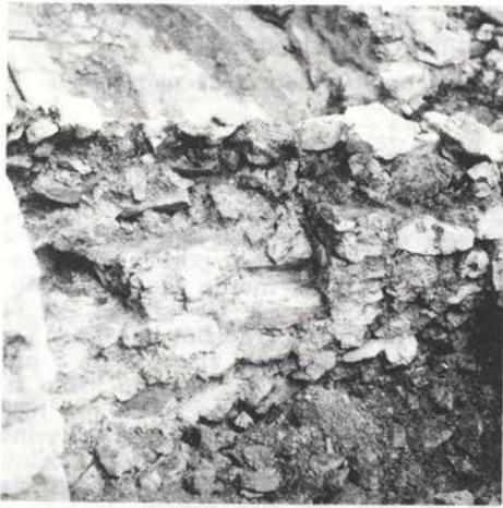
Sl. 77. Ajdna — zazidan prehod med obema stranskima prostoroma Fig. 77 — Ajdna — walled-in passage between both side-rooms
