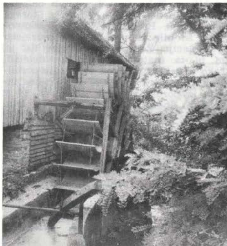
Sl. 10. a, b: Polže — pogonsko kolo žage venecijanke med in po obnovi Fig. 10 — a, b: Polže — driving-wheel of a Venetian saw during and after restoration
