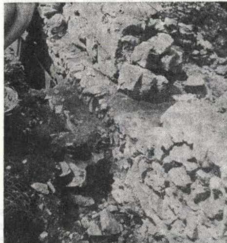
Sl. 25. Ajdna — Z ožjim zidom zazidan prvotni vhod in nadzidan del zahodne stene Fig. 25 — Ajdna — original entrance walled-in by a narrower wall and the above built part of the western wall
