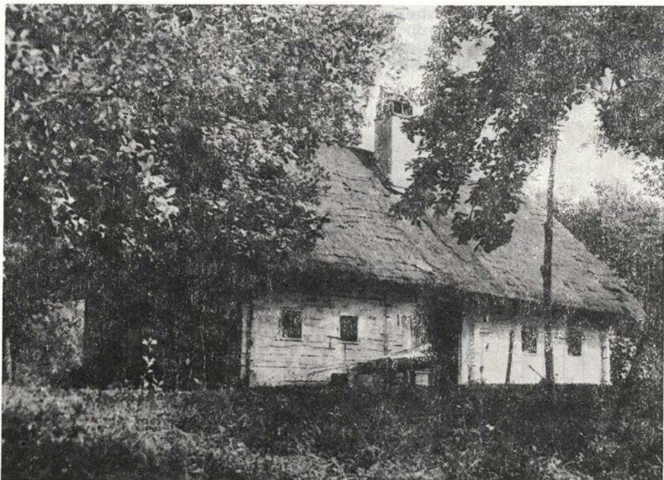
Sl. 102. Poklek 22. Stanovanjska hiša, ki jo je lastnik porušil maja 1987 Fig. 102 — Poklek 22. Family house pulled down by the owner in May 1987
