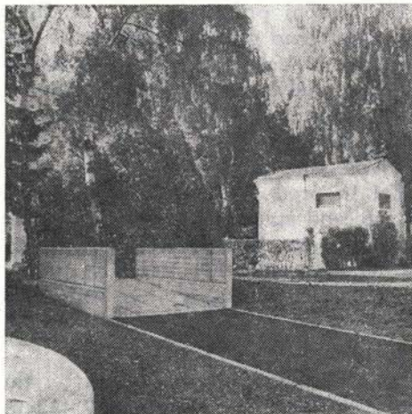
Sl. 81. Betonske ograje ob vhodih Fig. 81 — Concrete fences flanking the entrances
