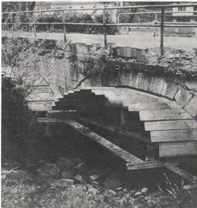
Sl. 97. Kamna gorica, sanacija kamnitega mostu Fig. 97 — Kamna gorica, sanation of the stone bridge
