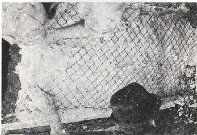
Sl. 35. Hajdina — odlivanje peči (3. faza): prekrivanje žičnega prepleta z mavcem (foto: Mira Gulič) Fig. 35 — Hajdina casting of the kiln (phases 3 and 4): the interweaving of wire being covered by plaster (photo Mira Gulič)
