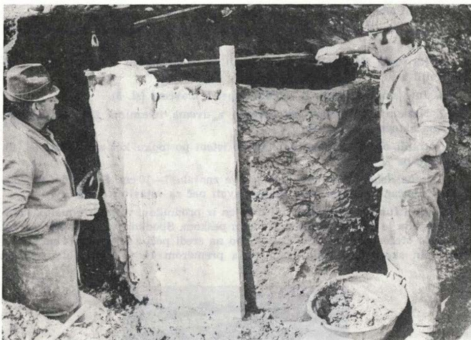
Sl. 34. Hajdina — odlivanje peči (2. faza): nanos plasti mavca na plast gline (foto: Mira Gulič) Fig. 34 — Hajdina — casting of the kiln (phase 2): a layer of plaster covers a layer of clay (photo Mira Gulič)
