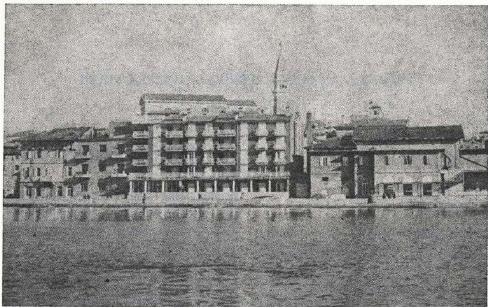
Sl. 79. Piran, del j. mestne fasade pred obnovo hotelskega kompleksa 1986 (J. Jeraša) Fig. 79 — Piran — the southern town façade after the interpolation of the new building in 1986 (photo Gale D.)
