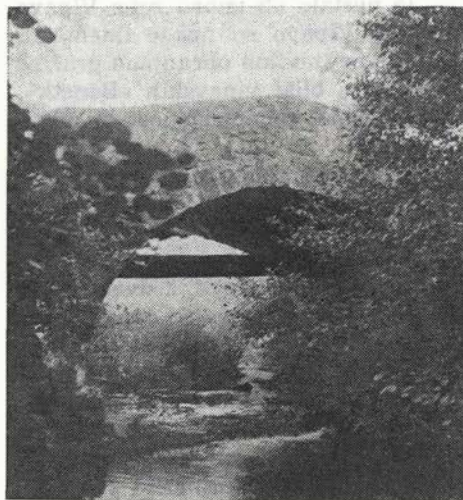
Sl. 121. Sela — most (Gorjup 1986) Fig. 121 — Sela — a bridge
