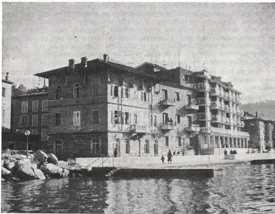
Sl. 82. Piran, j. fasada hotela pred prenovo (J. Jeraša) Fig. 82 — Piran — the southern façade of the hotel before the renewal (photo J. Jeraša)
