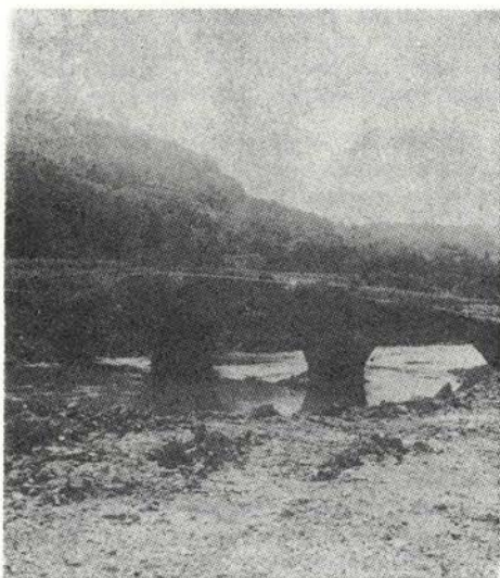
Sl. 135. Dolenje, kamniti most s tremi loki Fig. 135 Dolenje — a stone bridge with three arches
