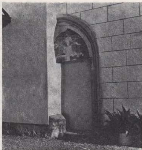
Sl. 12. Lesce — zazidani zahodni portal zgodnjegotske cerkve s fresko v timpanonu Fig. 12 Lesce — walled up west portal of the early Gothic church with a fresco in the tympanum
