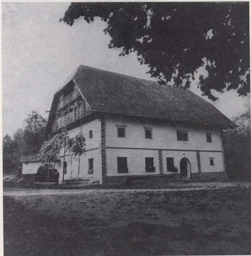
Sl. 136. Podbrezje št. 18. Zidana nadstropna hiša po obnovi fasad l. 1984, restavrator T. Marolt Fig. 136 Podbrezje no. 18. Stone-built storeyed house after the restoration of the facades in 1984, restored by T. Marolt
