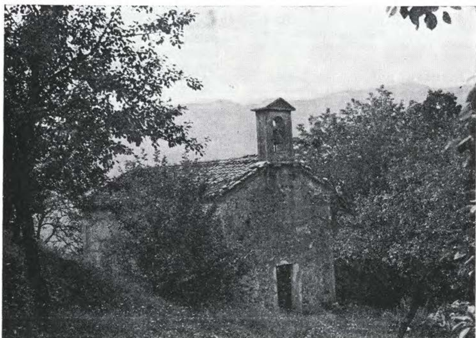
Sl. 121. Koseč — cerkev pred obnovo Fig. 121 Koseč — church before the renewal
