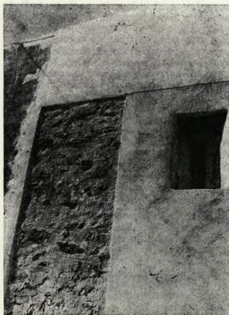
Sl. Svibno, ž. c. sv. Križa. Prezentirana romanska zidava ob zgodnjegotskem okencu Fig. 103 Svibno, the parish church of St. Cross. The presented Romanesque building remnants by the Early-Gothic window
