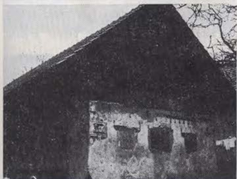
Fig. 4-6 Leskovec above Višnja gora. House No. 2 before and (below) after the restoration; on the right: a detail. (Photo: A. Bar-Janša)
