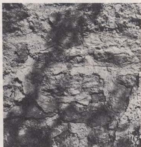
Fig. 7-9 A part of the south wall of the church's aisle, with a Romanesque small window and four plasterings; a characteristic construction of the south wall of the aisle
