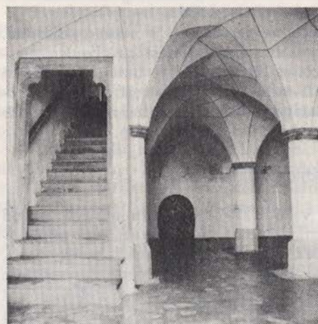
Fig. 8–10 Restoring the groundfloor: removal of structural alteration, deficient in quality, (right) the uncovered system of the reticulated painted vaults, and the restored hall-room and staircase
