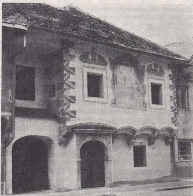
Fig. 19-20 The Sivec House prior to conservation works, in 1974; below: its presented façade, in May, 1975.
