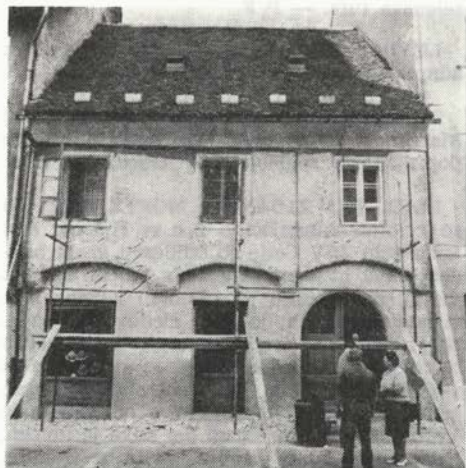
Fig. 27—28 Kranj, Uncovering the original polychromy on the facade of the house at 12 Tito Square, and (right) the facade with the renewed polychromy
