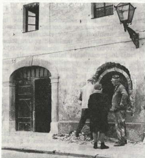
Fig. 22—23 Kamnik, Brigand's house prior to its adaptation, and (below) removing the original apertures
