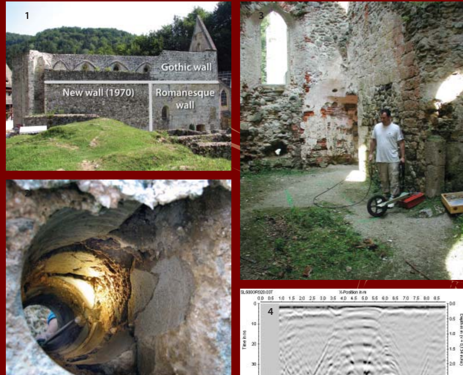
1. Different types of masonry at north wall, 2. Boroscopy investigation, 3. Non-destructive assessment of ground of the Otokar Chapel, 4. Radar traces of grave in the Otokar Chapel
